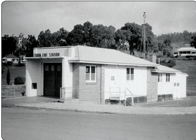
Bridgetown Fire Station. BHS 10-414
