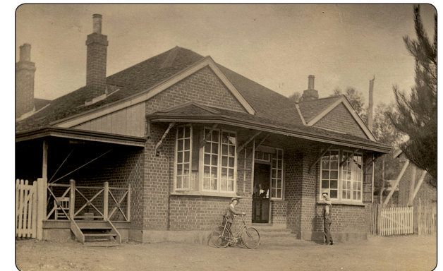
Original Post Office. BHS 95-253
